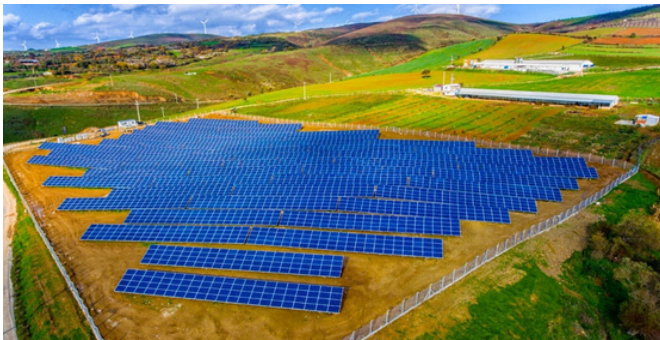
Solar Panel Project
