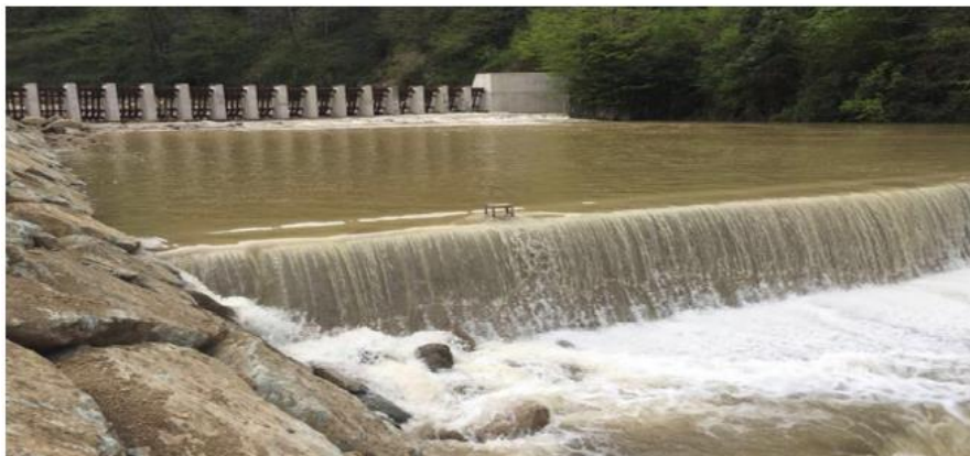
Figure 18. Permeable Sediment Collection Weir
