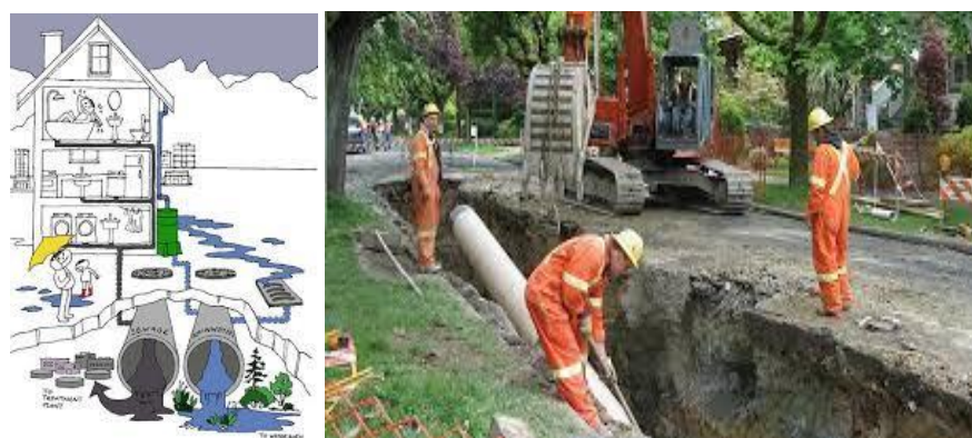
Figure 27. Separating rainwater from the sewer system
