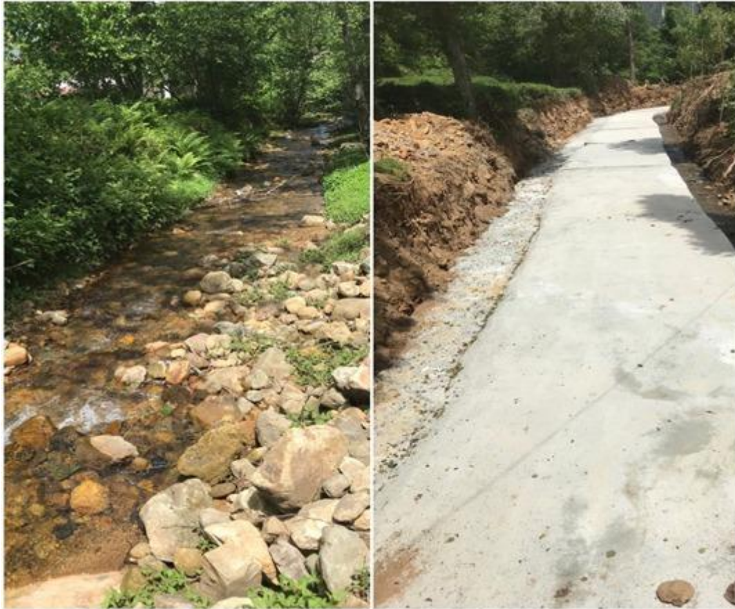
Figure 31. Stream improvement work by embedding in concrete.
