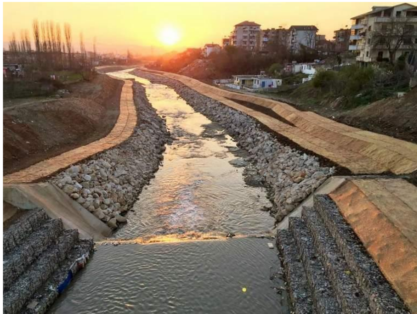
Figure 20. Stream channel Embankments
