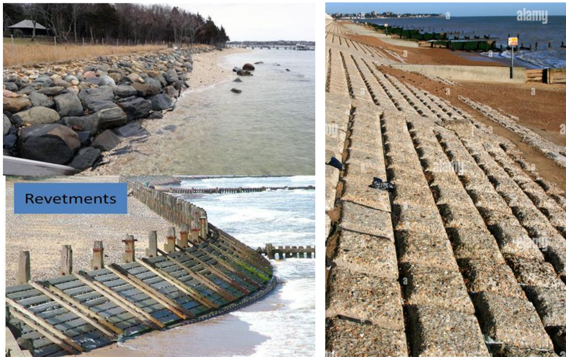
Figure 36. Examples of shoring or coatings (revetments)
