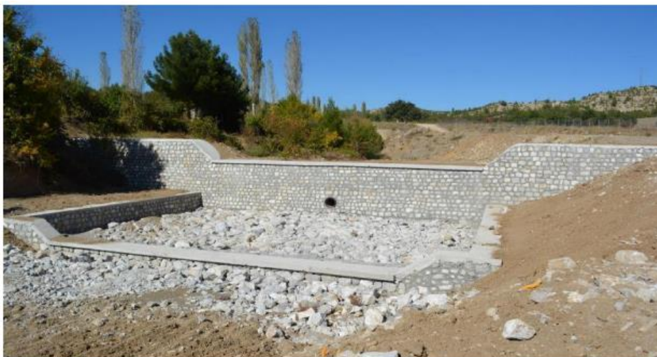
Figure 17. Example of a Sediment Collection Weir built upstream to contain excess sediment.
