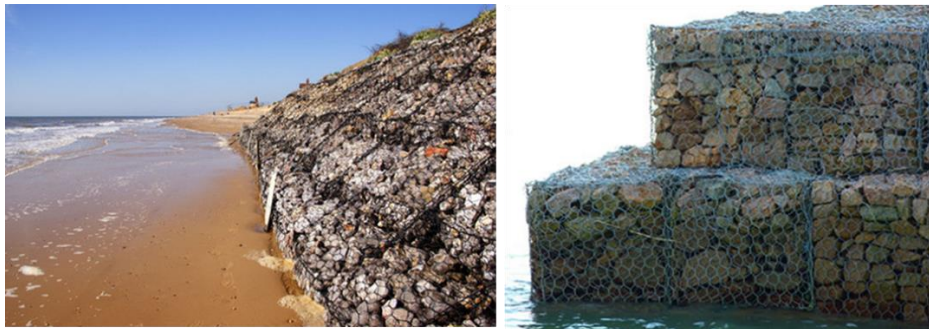
Figure 39. View of various Gabion structures on the shore.
