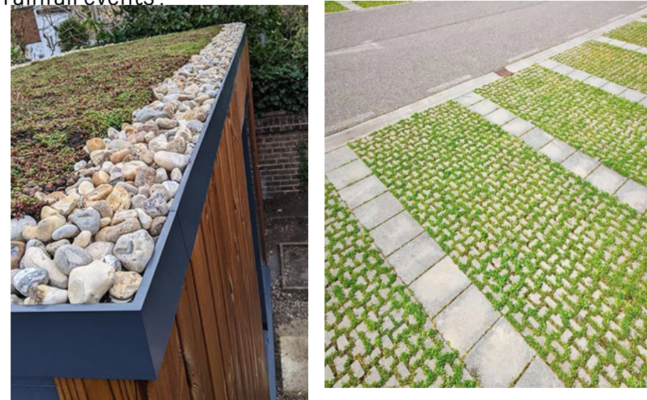
Figure X. Green Roof and water retaining pavement
